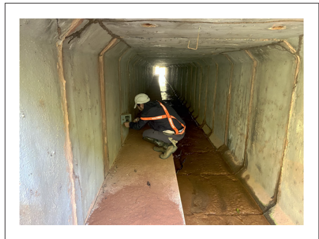
FIGURE 2. Highway underpass structure, camera trap position and installation.
